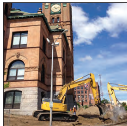
Brockton's City Hall Plaza Reconstruction project is underway
