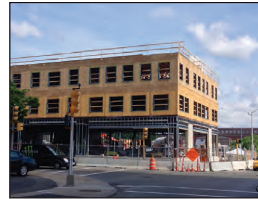
Construction continues on the Enterprise Block project in downtown Brockton
