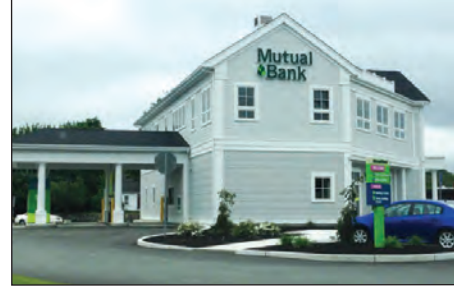
Mutual Bank's new 5600 square foot, two-story location in Whitman houses a full-service retail branch and offices for Residential Lending
