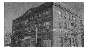
Photo of the completed facade at 278 Main Street, Brockton
