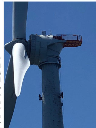
(Right) Regular painting and maintenance of the wind turbines are conducted to keep them ready for generating power
