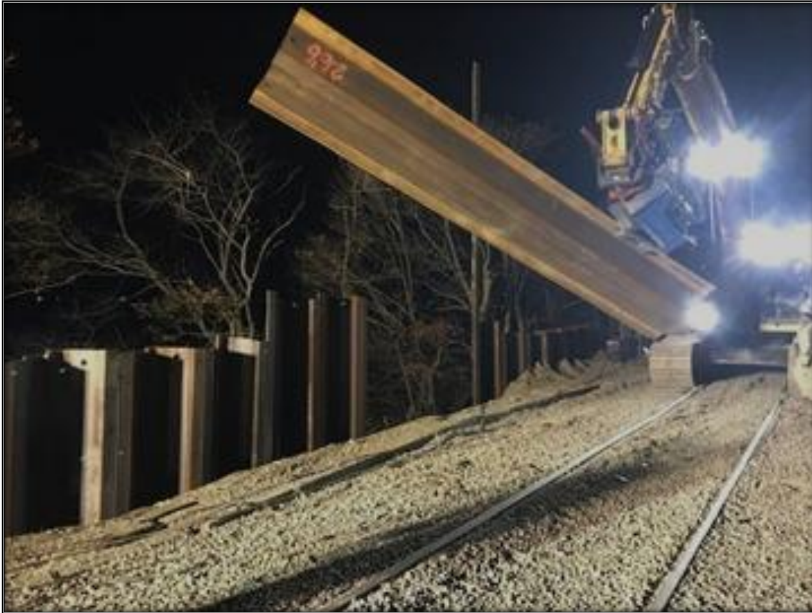
Installation of sheet piles
