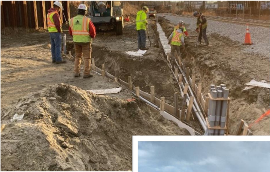
View of signal conduit routing
