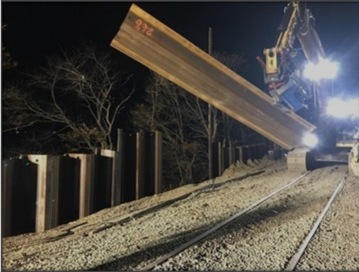
Installation of sheet piles
